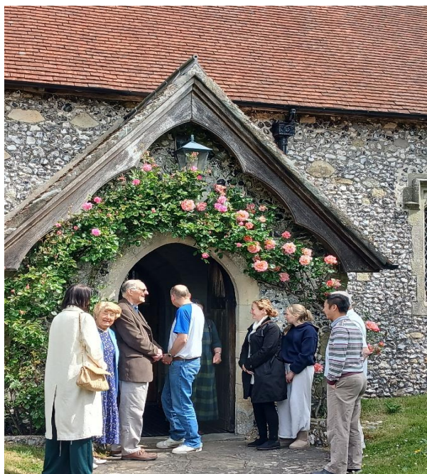
The main entrance to East Dean Church
